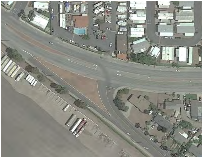
Image 1: La Verne Avenue & Arrow Highway Intersection
