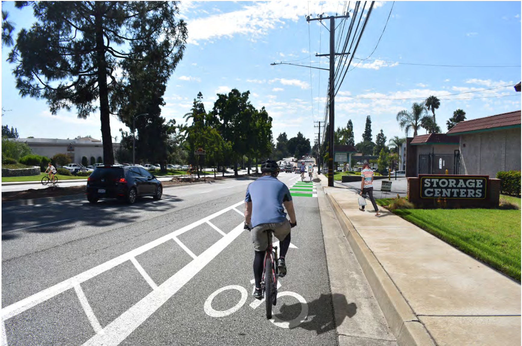
Figure 32: Rendering of proposed Class II buffered bike lanes between San Dimas Avenue and Walnut Avenue.
