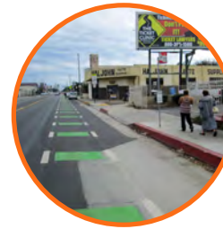
COLOR PAVEMENT TREATMENT Green Conflict Striping
