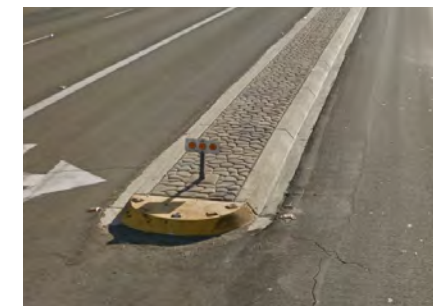
Concrete separator for access management (2')
