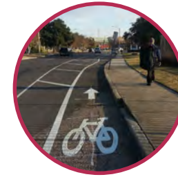
CLASS IIB Buffered Bicycle Lane
