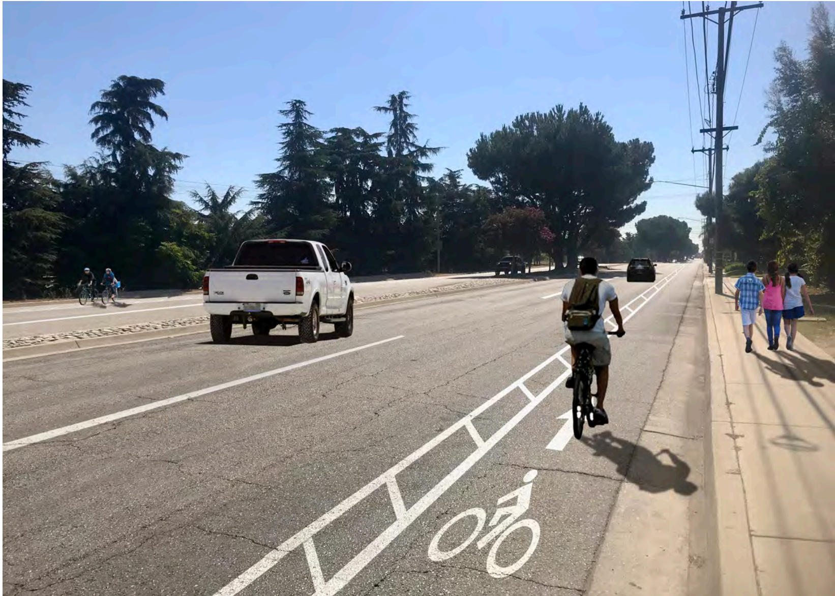
Figure 33: Rendering of buffered bike lanes along Arrow Highway between Park Avenue and A Street.
